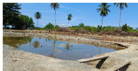
Figure 8. Swimming Pool Source: Research Data (2024)
